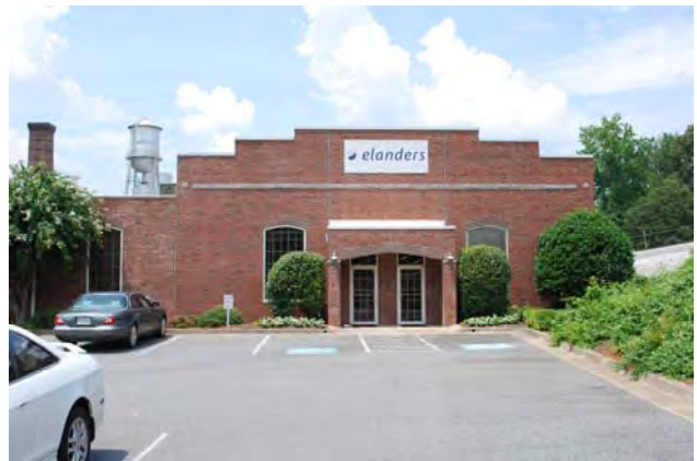
Photograph 002 Westerly View of Front (East) Façade Resource #1: Acworth Mill, Main Building
