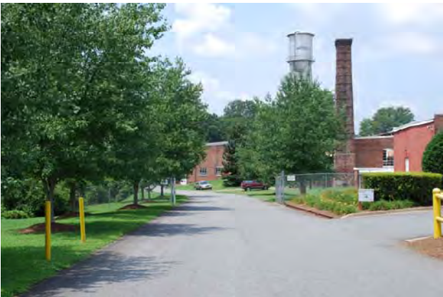
Photograph 057 Westerly View Along Existing Drive Behind Acworth Mill (Pelham Drive)
