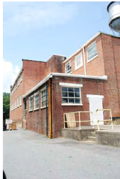
Photograph 058 Northwesterly Contextual View of Rear (South) Side of Acworth Mill Facility
