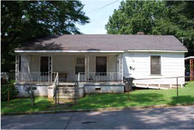
Photograph 011 Westerly View of Front (East) Facade Resource #12
