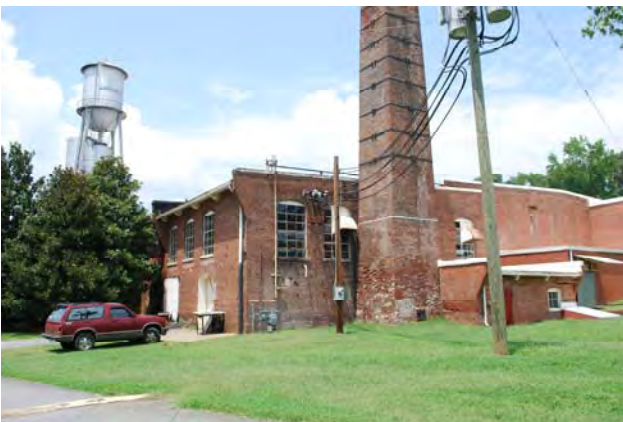
Photograph 003 Northwesterly View of Resource #2: Acworth Mill, Warehouse
