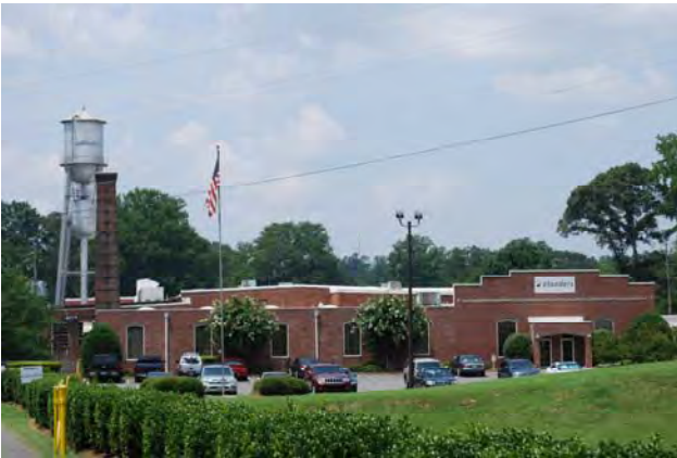
Photograph 001 Northwesterly View Toward Acworth Mill And Warehouse Buildings (Resource #1 and #2)
