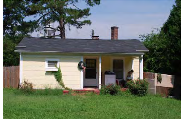
Photograph 038 Westerly View of Front (East) Facade Resource #58
