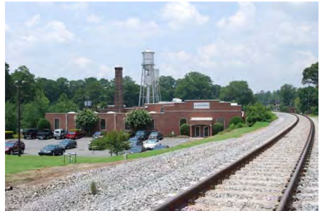
Photograph 040 Southwesterly Contextual View Along CSX Railroad toward Acworth Mill Facility
