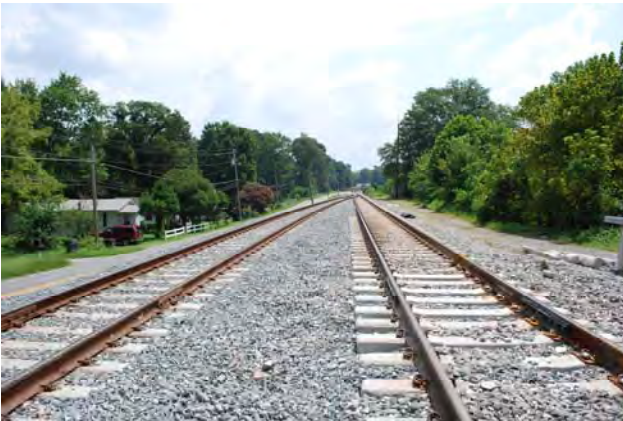
Photograph 039 Easterly View Along CSX Railroad Corridor Resource #59
