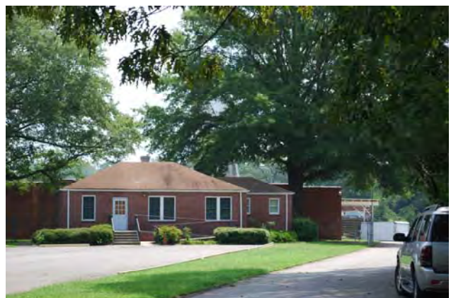
Photograph 004 Easterly View Toward Resource #3: Acworth Mill, Office Building
