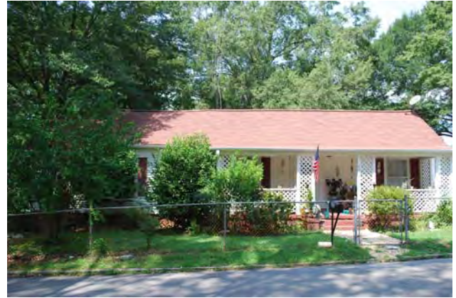
Photograph 012 Westerly View of Front (East) Facade Resource #14
